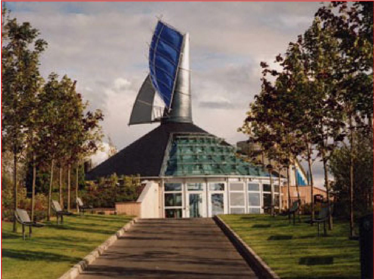
Figuur 14.6 - ICI Chemicals Visitor Centre Runcorn UK
