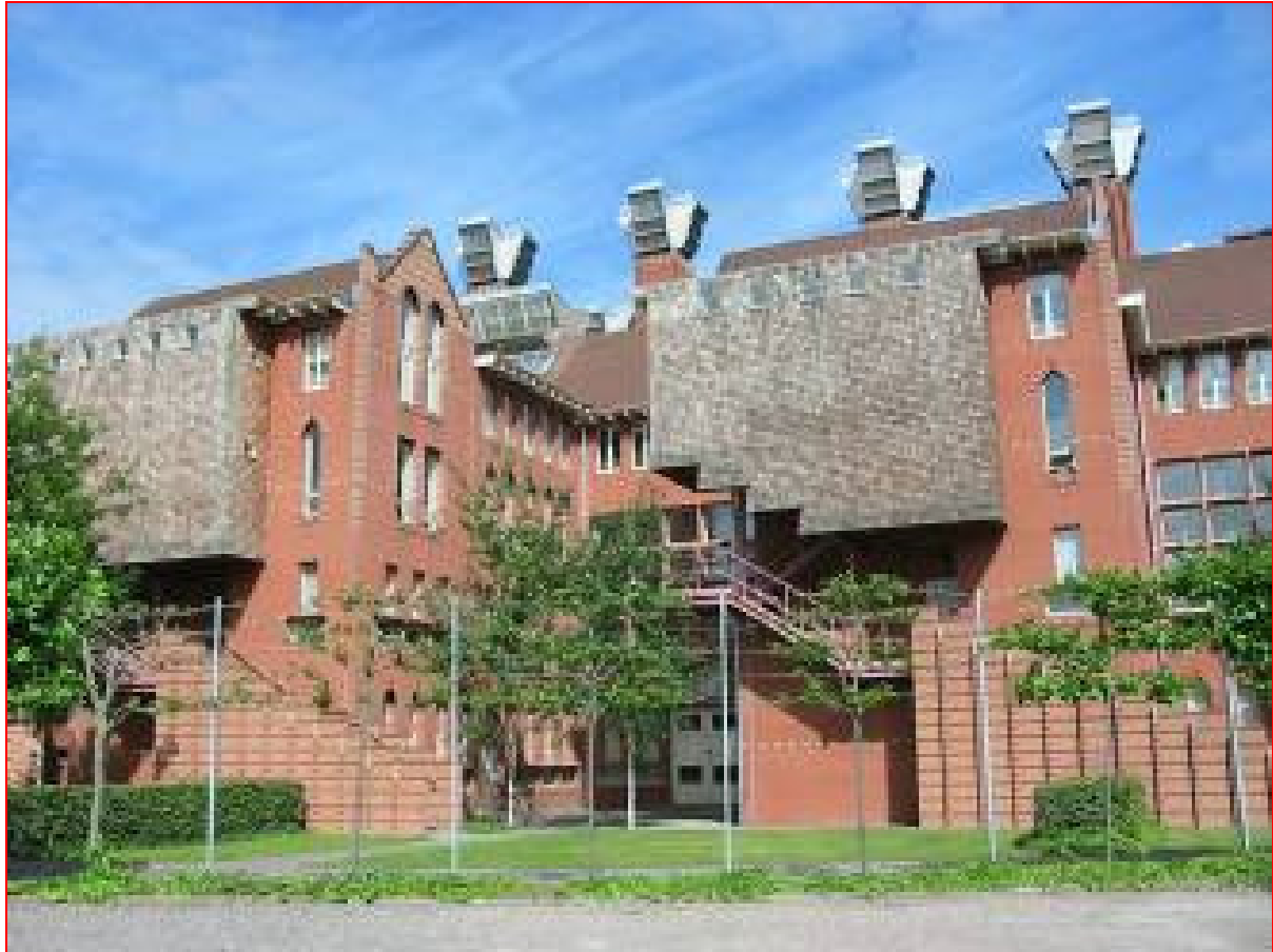
Figuur 14.11 – Queens Building De Montfort University
